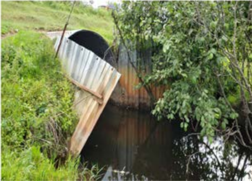
Culvert in Poor Condition
